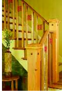
FAR LEFT: The house nestles into the wooded hill and is only visible as visitors make their way down a stony path. The Leifers didn't want to see or hear the road, so they sited the home below the street. Siding made from cedar shake and Maritek, a recycled wood composite, form the exterior facade. NEAR LEFT: The stairs are built using four different woods, including mahogany, locally grown and milled fir for newels, and local poplar and birch.
